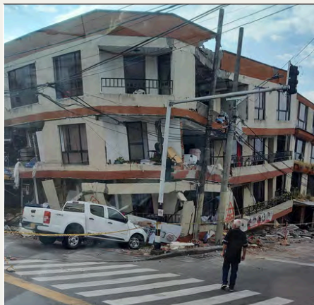
Buildings to be demolished
